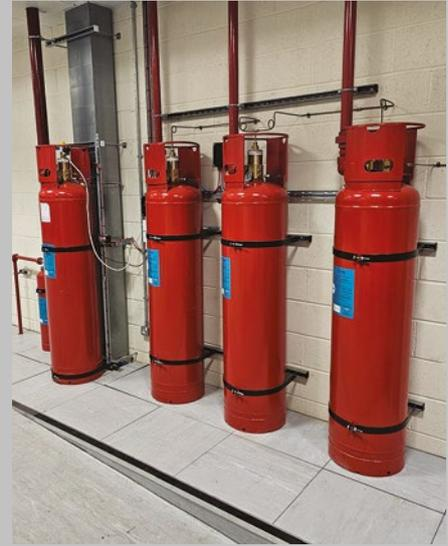
CRAC units removed and gas suppression bottles relocated to single location, freeing up floor space.
